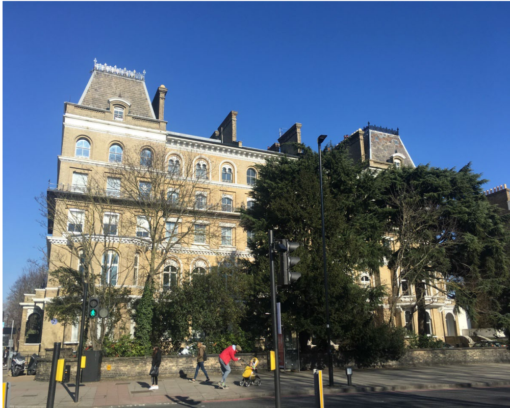
Figure 4.5: View of Cedars Terraces, a mansion block of 1860 overlooking the Common
