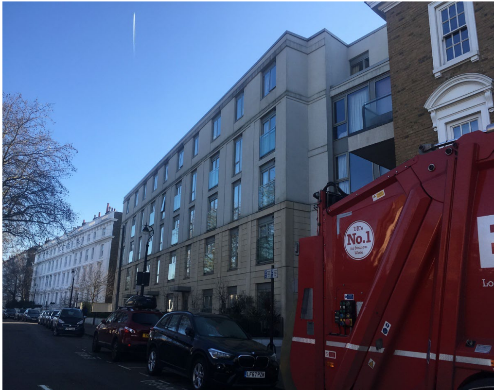
Figure 4.7: View along Grafton Square showing Wingate Square, a development from 2009
