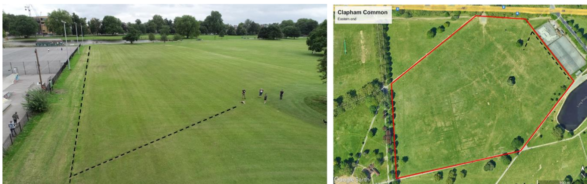
Figure 2-5 Drain lines incorporated and, R, their approximate location
