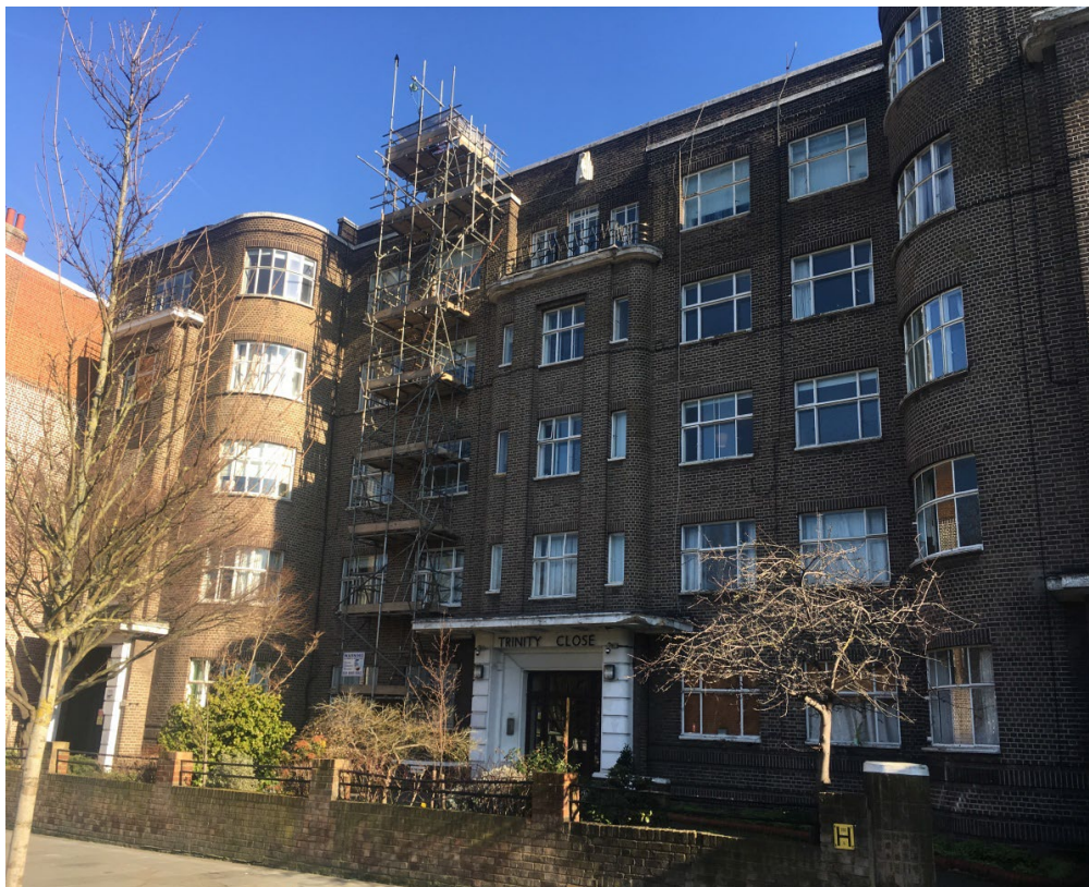
Figure 5.6: View of Trinity Close, an apartment building of 1936
